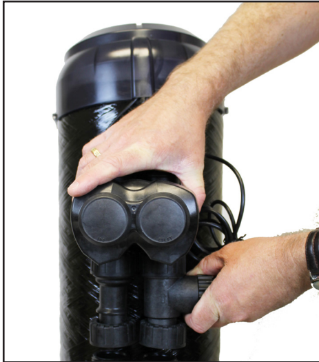
Attach water meter, spacer and bypass assembly. Lubricate connector O-rings with a food grade silicone before installing on bypass. HAND TIGHTEN ONLY!
