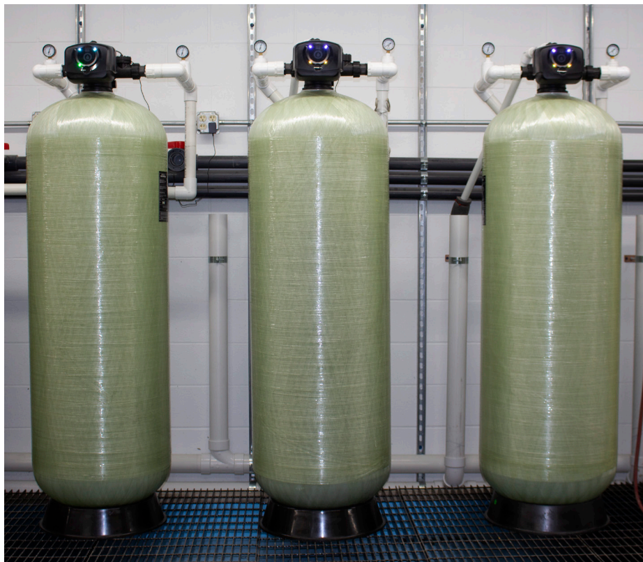
Commercial Triplex Softener System using DROP 1.5" Valves
